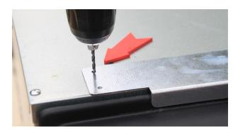
Mark and fix the top retaining bracket so that it holds the plenum box flange. not too tight but enough to hold a seal against the filter
